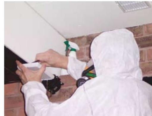
Externally, boarding around the roof line are common examples of cement based products which may contain asbestos if they were installed before the end of 1999.
